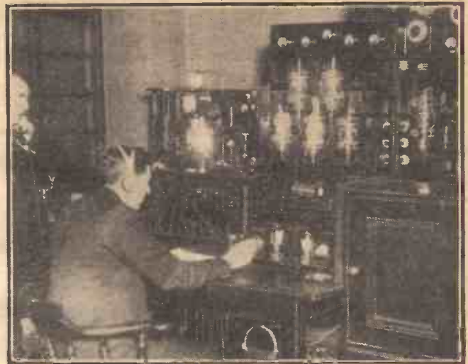
Sheffield—the first relay station in this country—will be closed down when Moorside Edge is in full blast. Here we see the Sheffield control-room.
