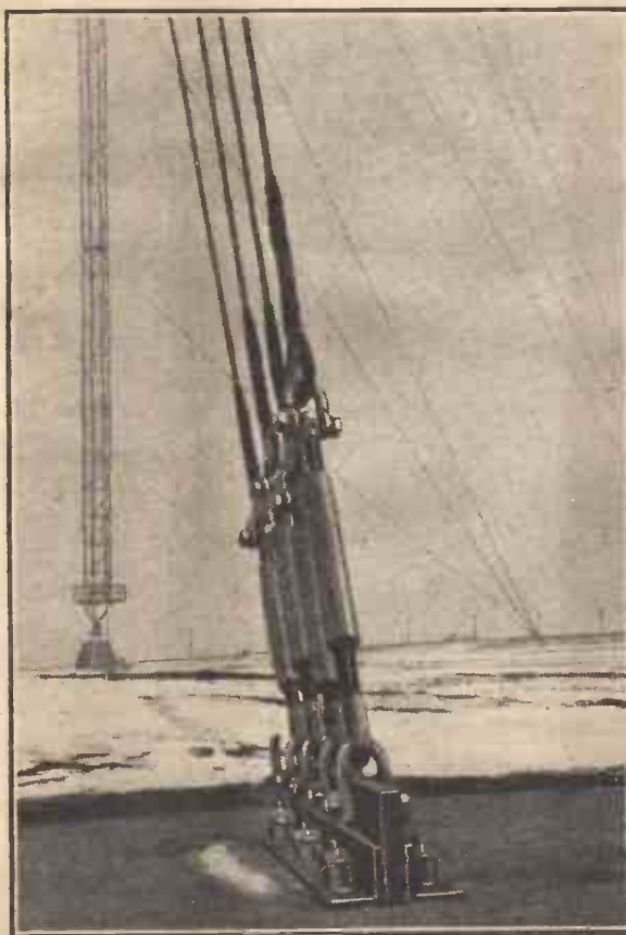
Gales blow with terrific force over Moorside Edge, so the mast stays have had to be anchored to massive concrete blocks let deep into the ground.
