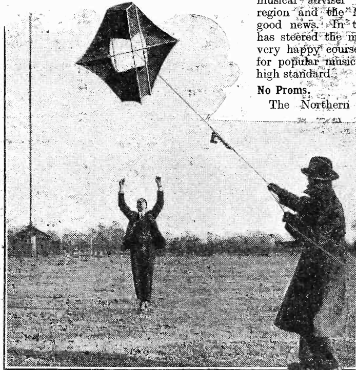
They are experimenting with kites carrying radio transmitters at the Slough Radio Research Station. They are one-valve transmitters using tiny cells for L.T. and H.T. and weighing less than a pound. The kite goes up to a height of about 500 feet, and 100 feet of the cable is aerial. A range of about one mile is achieved.
