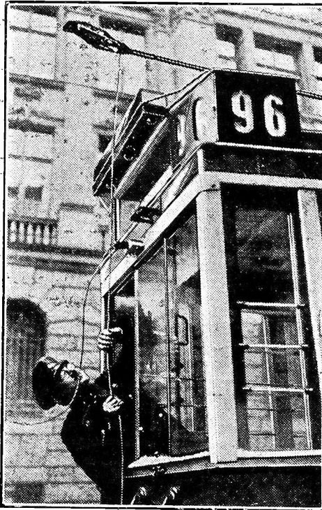
Trying out a new German device for the elimination of radio interference caused by sparking trolley-poles on tramcars. It consists of a scheme that bypasses the spark energy to earth, thereby preventing the spark forming.
