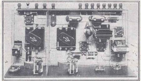
Contrast this view of a modern receiver—the "Regional" Four—with the photograph of an old-tashioned set on the preceding page. Well-spaced wiring is necessary if the selectivity of several stages is to be retained.
