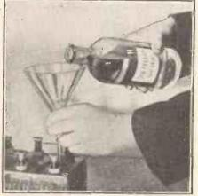
Topping up the accumulator with distilled water should be done regularly.
