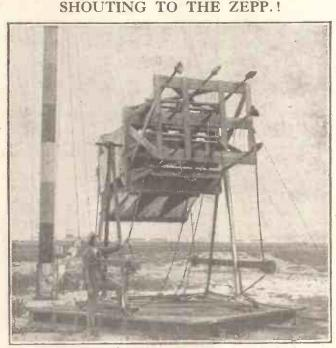
This is the giant loud speaker used at Lakeburst, N.J., to shout directions at the "Graf Zeppelin" in its landing operations.
