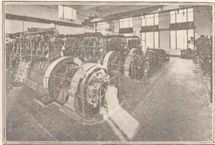
This is the power-house in which are the four Diesel engines and the dynamos for providing electric power for the whole station.
