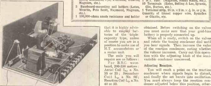
Careful spacing of components and neat wiring go a long way towards ensuring an efficient receiver.
