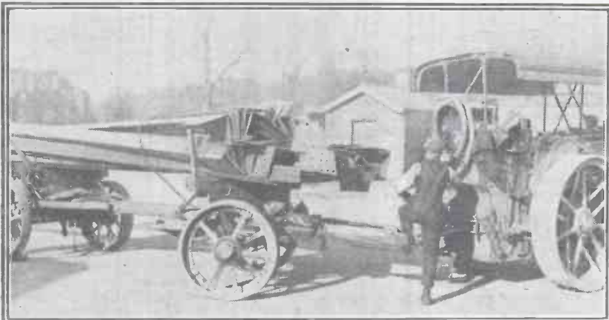
This photograph shows some of the steel girders for the aerial masts arriving at the new London Regional station, near Potters Bar, Middlesex.
