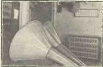
Two of the original loud speakers—installed in 1896—still used for checking purposes at the transmitting station.
