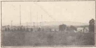
The tall masts at Klipheuval are being abandoned in favour of the short ones also shown, now that the Beam is to be used.
