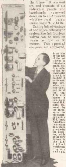
one for short waves and the other for the "broadcast band" (300 to 600 metres). Thus the whole sot operates efficiently on the low waves with the super-het. unit in circuit, and, with this removed, the receiver is a long-wave twelve-valver, capable of handling wave-lengths between the hundreds and the tens of thousands.
