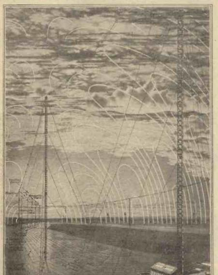
This picture illustrates the manner in which ether waves are caused to radiate from the great Rugby station aerial system.
