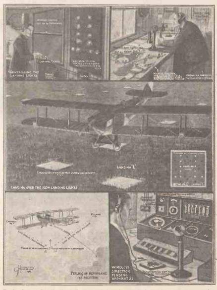
Showing how wireless direction-finding apparatus is used to check the positions of aeroplanes during flight. Information respecting landing lights, etc., can also be conveyed by radio to the machines.
