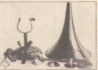
The complete set of parts used in the home constructed loud speaker.
