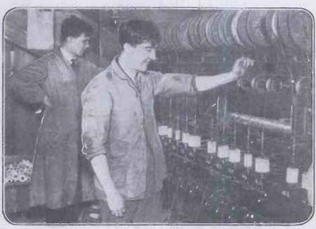
Covering wire with silk and cotton insulating material in a large wireless works at Acton.
