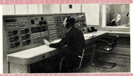
More unitidous is the new Control Room as Back House fonding which handles programmes for BBC's Overseas and European Services. The vaupment designed by BBC engineers provides removely controlled witching for the connection of 150 sources to 112 outgoing routes. Programmes in the Overseas and European Services total nurse than 82 hours a day
