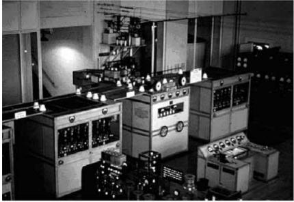
Picture 10: One of the original twin transmitters at Brookmans Park, with 2LO in the foreground, c1970
