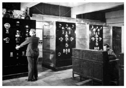
Picture 6: Sender 1, one of the two original short wave transmitters installed in 1932 at Daventry Empire Station, c1942
