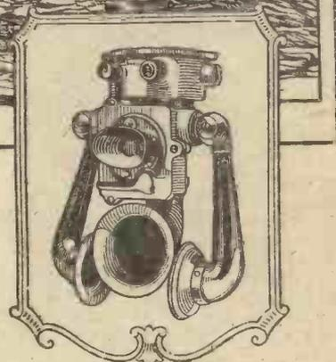
A typical Graham Loud Speaking Naval Telephone, as fitted on board ships of the Royal Navy.
