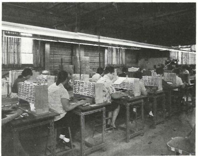
Production line splicing section of the Stereodyne factory/warehouse/office complex.
