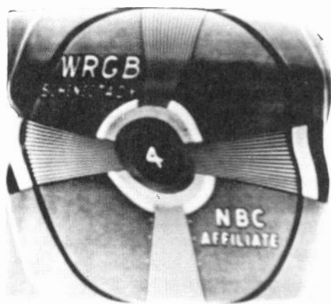
Fig 5-D. Distortion due to hum voltage
