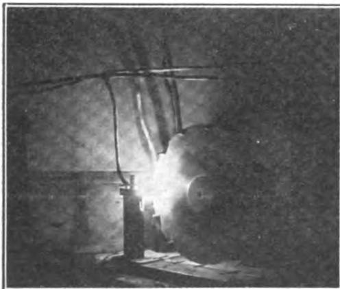
*Siasconset's spark. This photograph was made with a 5 sec. exposure while the disc was running at 1800 R. P. M. Although traveling at a speed of more than 100 miles an hour, the studs appear to be standing still, due to the fact that the disc was illuminated only at the instant when the moving stud came opposite the stationary stud, causing the spark to discharge.*
