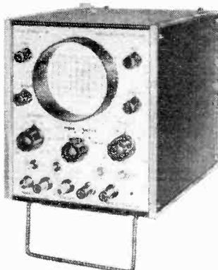
Bradley transistor oscilloscope. Tube is 3in diameter.
