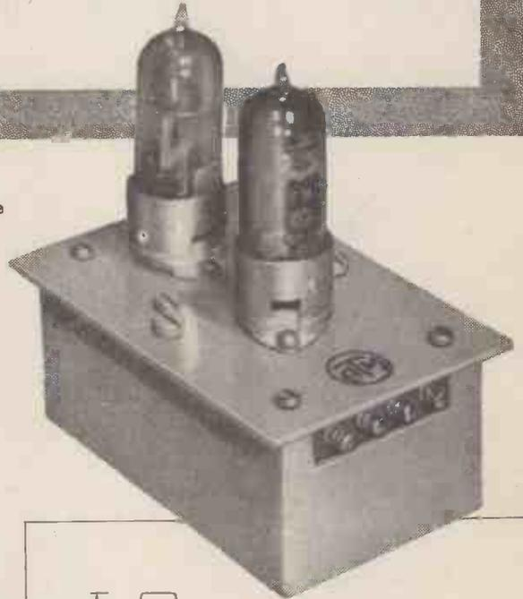
This crystal oscillator has been designed by A.T.E. to overcome the disadvantages of oscillators of the oven mounting type in situations where immediate operational availability is called for, i.e. transport and defence requirements. The unit has the advantages also of great compactness, very simple design and static components.
