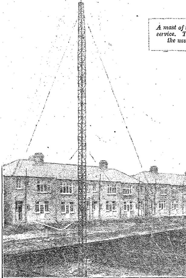
One of the masts at the station of Mr. F. H. Haynes (2DY). It is built to the design given in this article though the height has been extended to 60 feet.
