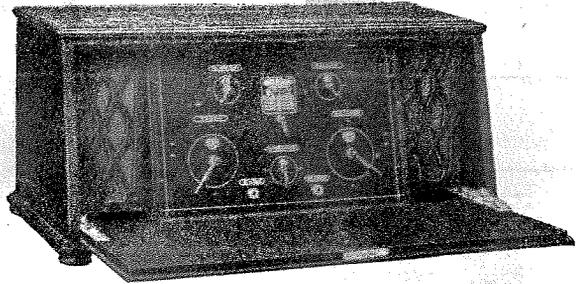
*A four-valve receiver by the Michigan Radio Corporation. This set has one stage of high frequency, detector, and two stages of low frequency amplification. The set is equipped with a self-contained loud speaker, and there is ample room for the batteries.*
