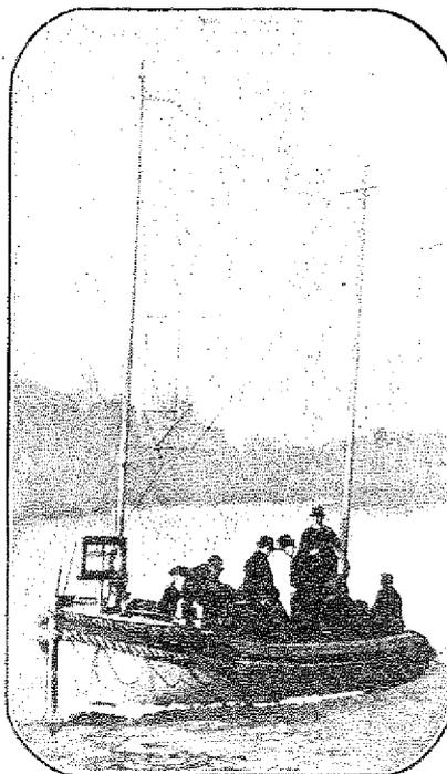
**SAFETY AT SEA.** One of the wireless-equipped lifeboats of the R.M.S. "Orbita," undergoing her tests at Liverpool. Note the D.F. frame in the bow.
