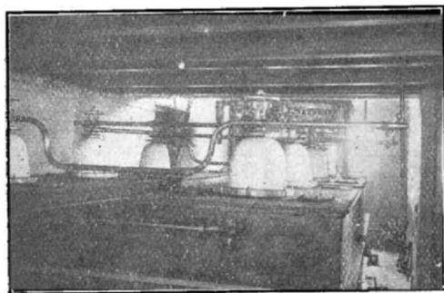
Fig. 4. The bank of four condenser units.
