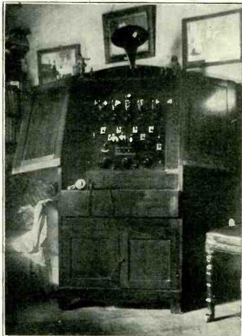
Our photo shows the five-valve receiver constructed by Mr. Arthur W. Botten, of "Red Cottage," Bourne End. By means of Dewar type switches, any combination of valves can be obtained. Compactness has been aimed at throughout, and the only visible wires are those to the phones or loud speaker.
