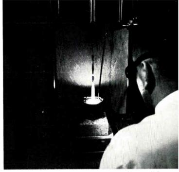
Neodymium in scheelite (calcium tungstate) crystal for an optical maser grown by Czochralski method at Bell Telephone Laboratories.
