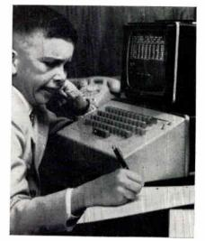
No cowboys and Indians here. Ten-year-old Wayne Burner tries hand at operating new General Electric Datanet-760 Keyboard Display Terminal. Device will display data stored in GE-235 computer systems. Device also allows changing and updating of data in the computer from the unit's keyboard.
