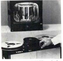
Precision Instrument PI-4V TV recorder features StopScan and VariScan, single controls which allow playback at stop-motion, or slow motion at any speed up to original recorded speed. First 23 of the 75-lb devices have gone to the Air Force for instructor training.
