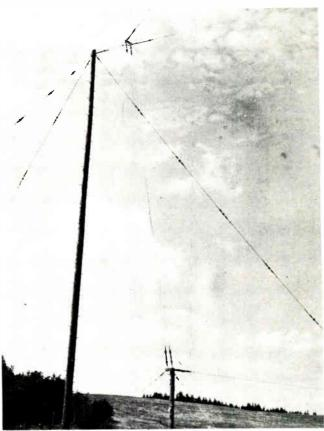
The input end of a common rhombic high frequency antenna.
