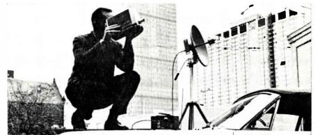
All-solid-state portable TV system introduced by Microwave Associates works from auto cigaret lighter. Works from 1.9 to 2.1 gc and mobile relay band. Applications include high-speed data sending, radar, telemetry, multi-channel TV. Usable to 50-mile radius.
