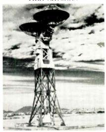
Above twin tracking antenna is one of two that Motorola built to test range and range-rate equipment it is making for NASA's Goddard Space Ctr. Twin antennas are at Motorola military test center, Scottsdale, Ariz. One "dish" transmits. One receives.
