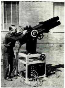
Optical photometer to detect presence of nuclear debris from high-altitude explosions is checked by Dr. E. Manring, of Geophysics Corp. of America, Bedford, Mass., developer of equipment. Rapid-response photometer observes and records fast intensity changes in four spectral regions simultaneously.
