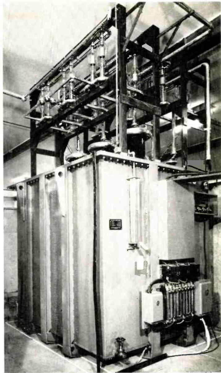
Fig. 3. 22-ton transformer for 150 kv 4.4 amp power supply.
