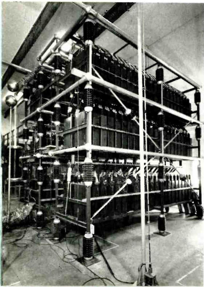
energy is that when an arc occurs in the final amplifier, something must be done to prevent the tube receiving all of the stored energy. Banks for use with electron tubes are now in design or operation at levels above 500,000 joules. 500,000 joules is the equivalent of  $\frac{1}{4}$  lb. of TNT. In view of this, perhaps the designer should be thinking about fault diverting equipment (commonly called crowbars).
