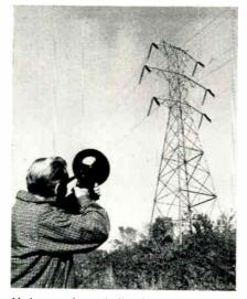
Aiming an ultrasonic "gun" at a high-voltage transmission line, W. E. Pakala of the Westinghouse research labs tests the line for electrical leakage, or corona. If present, corona produces high-frequency sound waves which are received by the "gun" and made audible through electronic circuitry. A telescopic rifle sight built into the instrument pinpoints the corona sources.
