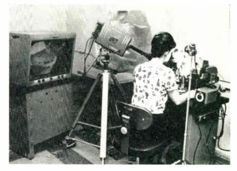
A closed circuit TV system is used by Kulicke and Soffa, Phila., to demonstrate how one of their machines operates in assembling a tiny transistor whose active area cannot be seen with the naked eye. TV equipment, made by the Dage Div. of Thompson Ramo Wooldridge, Michigan City, Ind. "sees" what the operator sees under the microscope and allows customers to observe on the monitor the moves of the precision machine. TV is also used for operator training.
