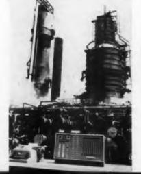
American Oil Co. has installed a fully automatic, closedloop, process control system developed by IBM at its 140,000barrel-a-day crude oil distillation unit, at Whiting, Ind. The control system which will continuously monitor and control the crude unit is built around an IBM 1720 Solid-State Digital computer.
