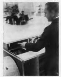
Eastern Air Lines ticket agent selects for viewing in a recessed monitor one of six channels carrying flight information at the new Atlanta Airport. Scan-a-graph System, designed and built by Nord Photocopy & Electronics Corp. of New Hyde Park, N. Y., transmits static information without vidicon camera or lights over coaxial cable.
