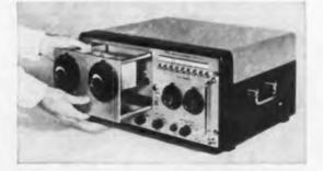
or production operations. Now, with one instrument and several, interchangeable plug-in oscillators, an engineer can cover a frequency range from audio to 3000 mc.
