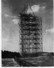
Saturn "dynamic test stand," in which the giant space vehicle's early three-stage flight model and second generation C-2 configuration will be assembled and tested, nears completion at the George C. Marshall Space Flight Center, Huntsville, Ala. The tower is 204 ft, high and incorporates some 600 tons of structural steel.
