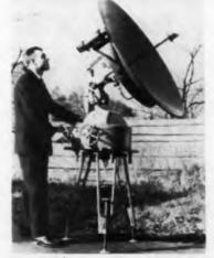
antenna for operation at 1680 MC  $\pm$  50 MC with gain of 22db over half wavelength dipole and 10<sup>\*</sup> beamwidth. Automation Dynamics is maker.
