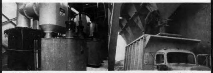
COMPACT HIGH VOLTAGE INSTALLATION. Westinghouse Silicon Rectifier Stacks are housed in Buell Transformer Rectification Unit (left rear). Tank (center foreground) is the separate Immersed Distribution High Voltage Switch Unit. An alternate Buell model encloses both units in a single tank.
