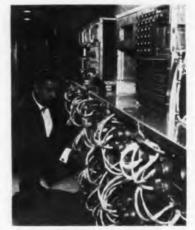
Missile monitoring station built into a Convair 240 twin-engine transport, "hears" and "talks" like a missile in flight, The planes have been converted into airborne stations for frequency monitoring and interference control (FMIC). Plane has 49 antennas, Engineer is William Garcia, Convair's project engineer,
