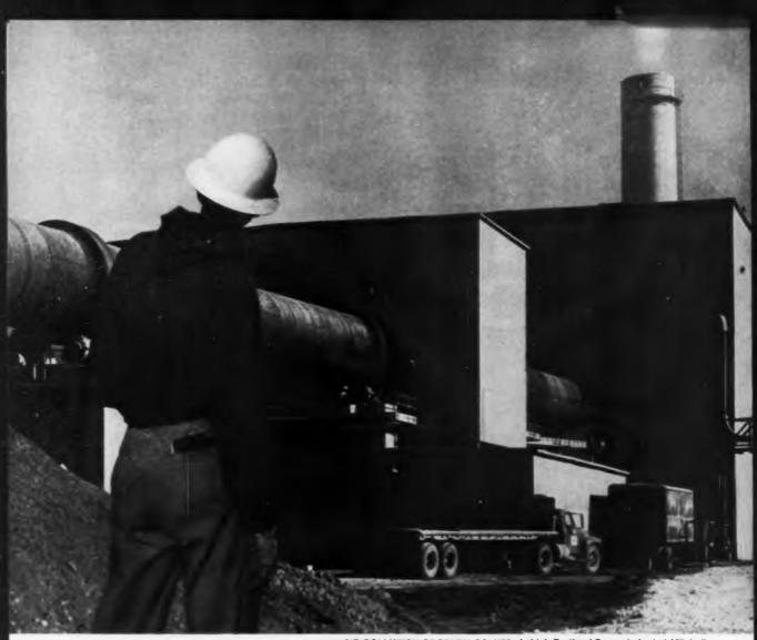
AIR POLLUTION PROBLEM SOLVED. Lehigh Portland Cement plant at Mitchell, Indiana, removes more than 99% of dust and impurities from kiln exhaust gases with four Buell Electrostatic Precipitators. Westinghouse Silicon Rectifier Stacks in the precipitators have operated without a single failure since installation in February, 1960. Rectifier units (in building above) <u>do not require</u> maintenance, temperature control, or ozone ventilation.
