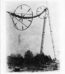
Seventy-four foot antenna insulator for the Navy's new radio station at Cutler, Maine, is tested on dummy tower at Lapp Insulator Co's, High Voltage Laboratory in LeRoy, N. Y. System will be used with Polaris FMB system.
