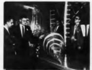
E. Blasi, P. Kennedy, Lenny Gatierrex, and R. Hoddle, Lockheed's Missile & Space Division, examine inflatable aluminum foil and plastic bag antennas designed for use with space vehicles. 6 psi is needed to inflate the antennas.
