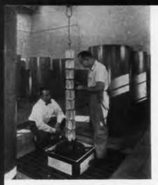
Synthetic crystals emerge from the growing vessel three weeks after being sealed inside.
