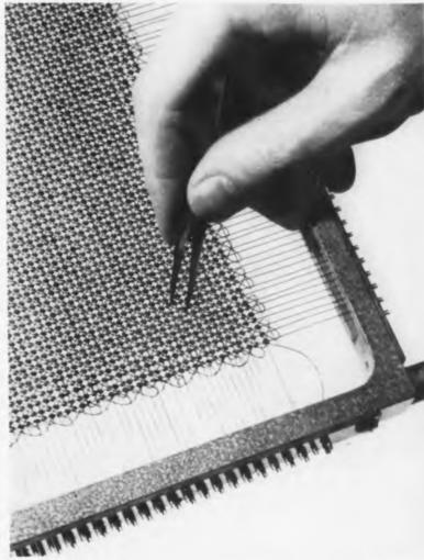
Over 1000 tiny magnetic cores strung on criss-cross wires less than 1 ft. sq. make up one unit of new magnetic memory in Whirlwind 1 digital computer developed at Mass. Institute of Technology. to provide Increased speed and reliability. It can take in or give out a piece of information in less than eight microseconds
