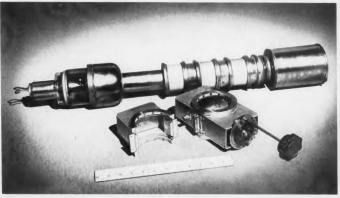
A power gain of 1000 times at 1200-1400mc in CW operation has been registered by the new Eimac X544 three cavity, cascade type klystron. With only three watts driving power the X544 delivers 3kw power output. This high power and high power gain is possible over a 200mc range through the exclusive Eimac feature of completing tuning circuitry external to the vacuum system. Other features of the Eimac X544 are a long life cathode, ceramic tube cavities, practical design and light weight.
