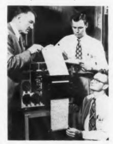
Fig. 5: Punched tape automatic sequence selector feeds flight plan data to controls
