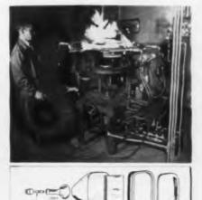
Faceplate of 24-in, Westinghouse color TV tube (top) is sealed to metal ring. Components of 70 tube with 200 sq. in. screen (bottom)
