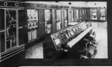
Transmitter room at WOR TV's new Empire State 50 KW transmitter, 130 KW ERP. 100°s air cooled. Completely sell contained. Equipment throughout by Standard Electronics.
