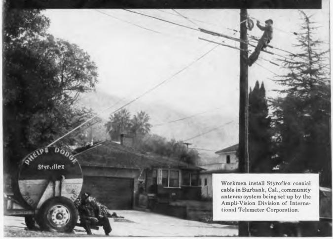
The superior operation, ease of installation, maintenance-free characteristics and low loss of Styroflex coaxial cable were proved in International Telemeter Corporation's first community antenna system at Palm Springs, Cal. This successful application has made Styroflex a unanimous choice for use in the company's second community antenna system being constructed at Burbank, Cal.
