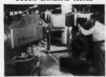
Color television cameras enter final test stage at RCA's Camden, N. J. plant, These initial commercial models are being shipped to networks and independent TV stations throughout the country
