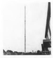
WHIO-TV, Dayton, Ohio, now has a 1104-foot TV tower in operation. The tower's builder, the Blaw-Knox Co., reports it to be the world's tallest. It weighs 600,000 lbs., is mounted on a 832,000-lb. concrete base, is 14-ft. triangular, and has an elevator to top
