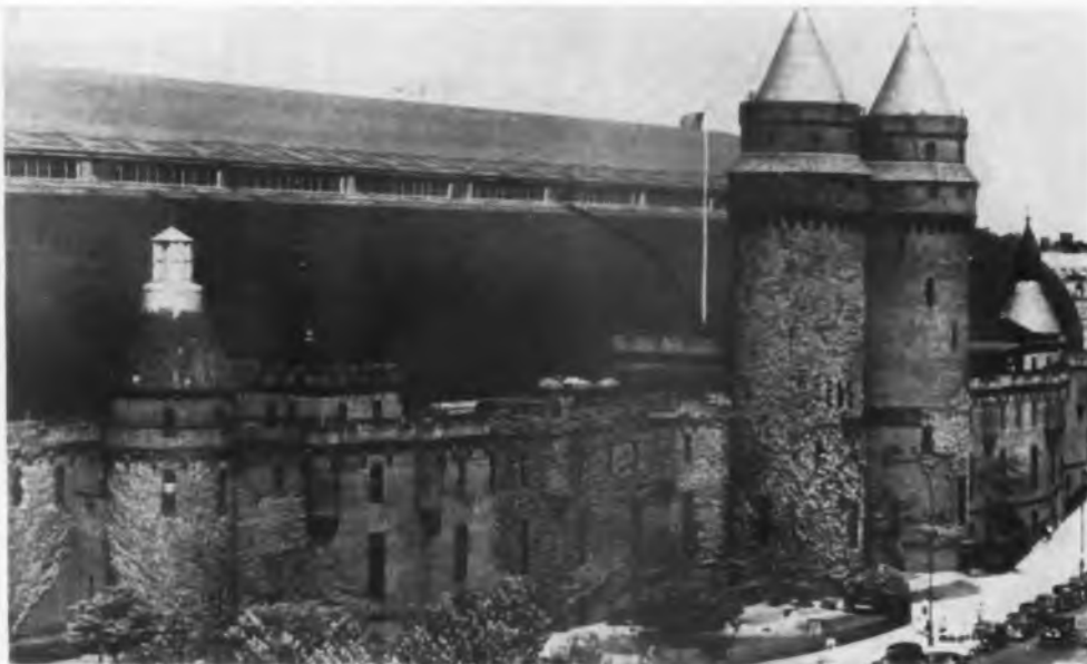
Kingsbridge Armory will house 3 meeting halls and 600 manufacturers' exhibits
