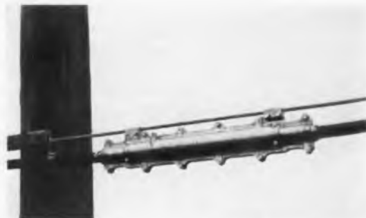
CLOSED CASING IN PLACE
