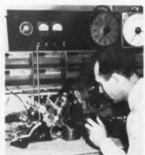
Fig. 4: Operator carefully observes etching of germanium for surface-barrier translator
