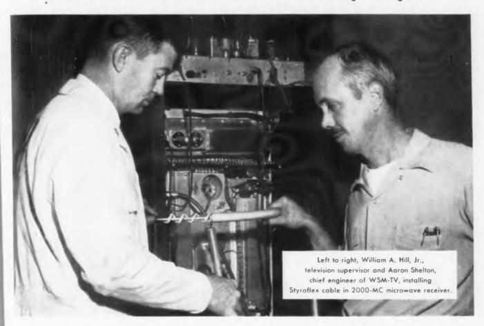
WSM-TV recently installed <sup>7</sup>s\* Styroflex coaxial cable feeding 2000-MC microwave receiver in local remote TV pickups. Chief engineer Aaron Shelton says, "We were able to gain better than 3 db, which we feel is the easiest and fastest and cheapest 3 db that we could possibly get!"
