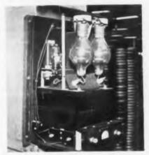
Electronic rectifier supplies dc to operate magnetic chucks in Nash production machinery. Electron tubes also control speed of maters
