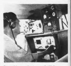
Magnecord tape recorder stores sounds picked up by microphones strategically located on moving car. Playback in laboratory will permit further analysis
