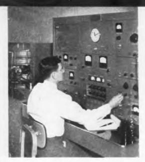
Research engineer makes a quantitive gas analysis on mass spectrometer at Ford Laboratory
