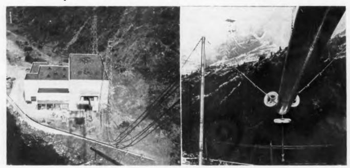
View of Navy's Radio Jim Creek transmitter building (1) from 200-ft, tower on summit ridge. Cables from span plunge down to tower of busing system nestled in valley between 3000-ft, mountains. View (r) from building housing world's most powerful transmitter shows antenna lead-in trunk and 145-ft, bus tower halfway up mountain which has been cleared of trees, "Doughnut" shields guard trunk from corona discharge, Official U.S. Navy photographs
