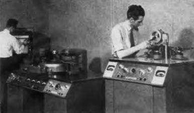
Cray diffraction film record (left) is scanned in microphotometer in GM lab. Beam is picked up on phototube, whose output is then ampified. Resulting signal is displayed on strip chart. In photo (right above) Engineer at left checks angular position on recorder of GE X-ray spectrogoniometer in Ford Scientific Laboratory. Researcher at right adjusts specimen position on X-ray diffraction camera
