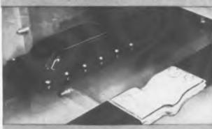
Expansion joint with and without Phenolite insulating covers
