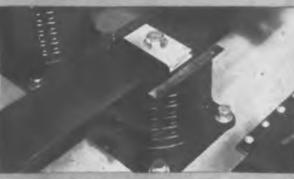
Bus support with and without Phenalite Insulating covers.
