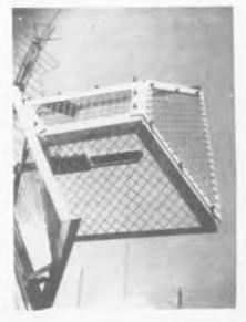
Fig. 5: WJZ-TV array consists of four corner reflector assemblies skewed around cone
