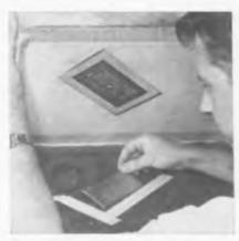
Fig. 6: Register guides are fastened to the printing base to locate successive base pieces
