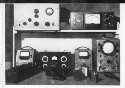
Fig. 1: Photograph of equipment employed to measure characteristics of iron-core transformers
