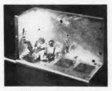
Fig. 10: Oscillator with special tube socket has minimum inductance and capacitance
