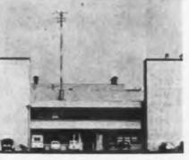
Pan American World Airways installation at Idlewild. Tower carries one 40 mc ground-plane antenna, six half-wave vertical 100 mc antennas, two weather instruments and a full set of obstruction lights.
