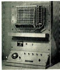
circuit with each of 100 sets of 6wire terminals, at speeds up to 50 sets per second. It is designed for fast, quiet operation without adjustment over millions of operations, with low crosstalk between adjacent circuits at frequencies up to 10 megacycles. James Cunningham, Son & Co., Inc., P. O. Box 516, Rochester 2, N. Y. Circle 357 on Inquiry Card. page 123
