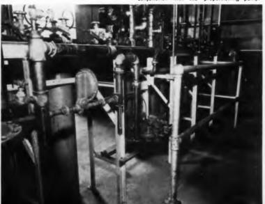
The actual plumbing which is used in conjunction with the proportioning pump.
