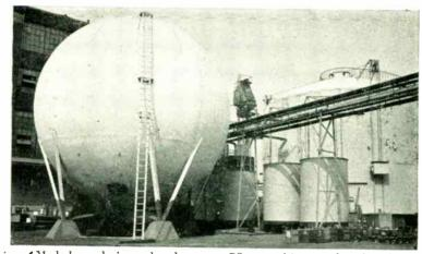
Made by exclusive carbonyl process: CO gas and iron ore form liquid iron penta carbonyl. Decomposed by heat into powdered iron, CO gas. Two unique results: chemically pure iron penta carbonyl and spherical iron powder particles. Photo above: Hortonsphere for storing CO under pressure.
