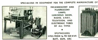
36 HEAD RADIO TUBE EXHAUST-ING MACHINE WITH BOMBARDER
