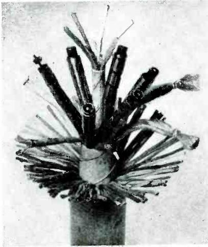
Bell Telephone six-coaxial cable. Included are a number of regular telephone wires
