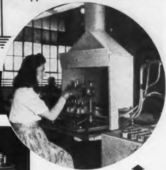
Electronic heater being used to solder on the covers of G-E capacitors. Four units are soldered simultaneously.
