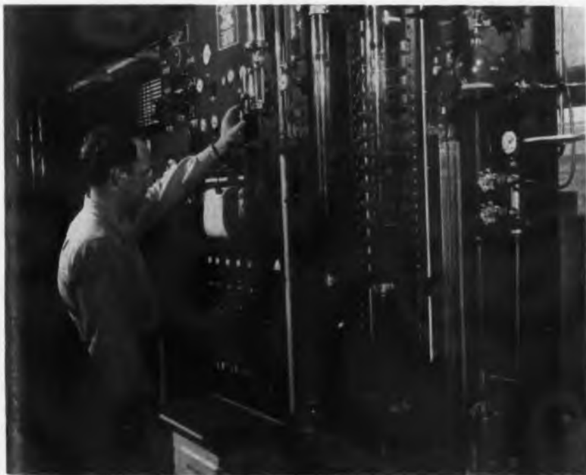
Electronic laboratory controls have been installed in the recently completed Richfield 100-plus octane refinery near Los Angeles. The unit pictured is a pilot fractionation tower that accurately determines the boiling point of any hydrocarbon fraction, enabling high efficiency separation
