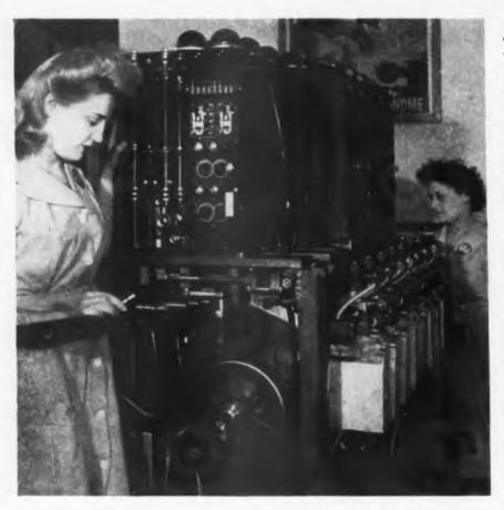
Shells are fed by hand into the dimension gage via an inclined chute. Cover removed from first photoelectric unit
