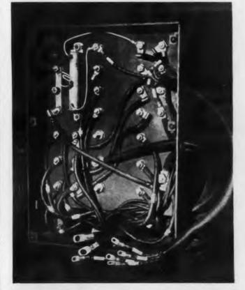
All connections in this panel on Diesel generating unit are made with Burndy Indent connectors, both the straight barrel and the right angle types being used.
