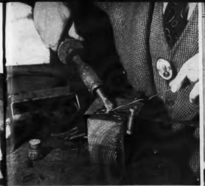
5. Above: Studies in chemical engineering developed several noteworthy wartime substitutes at RCA Victor Division, Camden, N. J. New "L-R" soldering flux overcame soldering problems, particularly with steel, which demanded fluxing agent more vigorous than rosin but less corrosive than sine chloride or other acids requiring water-washing. L-R flux is mixture of rosin and levulinic acid (corn starch derivative)
