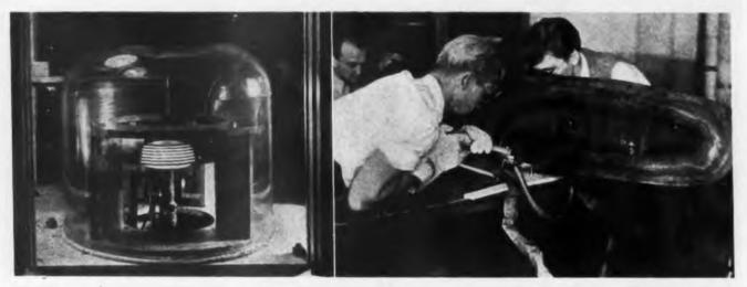
Oil well rock bit (red-hot) being hardened in experimental Westinghouse induction heating furnace. (Right) brazing a filet along the inside edge of hollow airplane propeller
