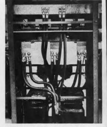
On this large rectifier unit all connections are of the permanent indent type. View shows only terminals; but Indent connectors are also available for and-to-ond as well as detachable connections.
