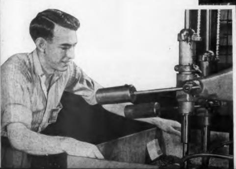
**1** \* STRIPPING enameled wires for soldering. New method at Electronic Laboratories, Indianapolis, Ind., is twice as fast as old way and lengthens life of wire brushes in motor-driven stripper. Solder pot at right, filled with molten lead, softens enamel before brushing.
