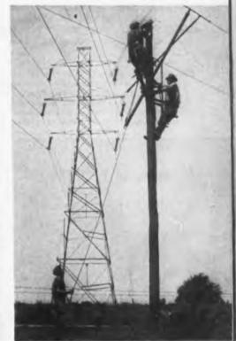
Fig. 6-Linemen, replacing insulator an 6.8 kv line, can be called in emergency by space radio
